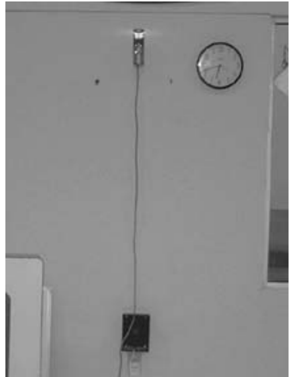
Figure 21.9. Light Tower Installed in the Adult Activity Center
