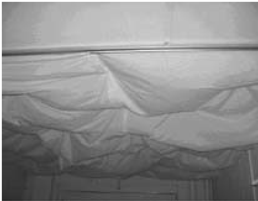
Figure 21.2. Ceiling with Fabric
